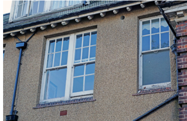
Joinery in need of repainting and bird spikes
