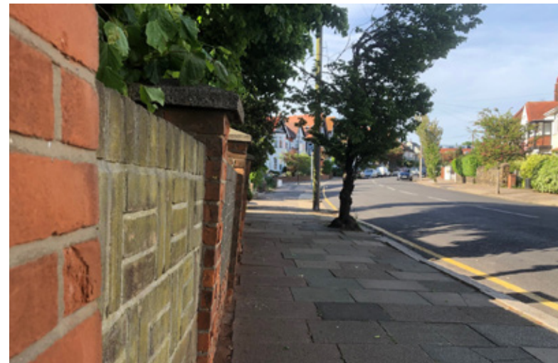
Boundary wall to Crowstone House which is leaning due to impact from tree roots
